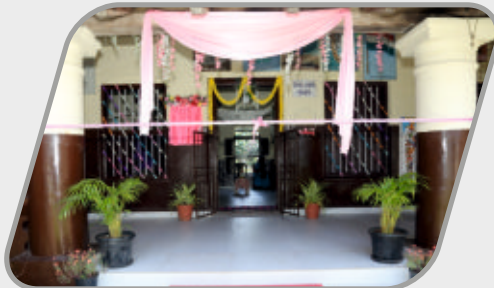
Primary School Renovation
